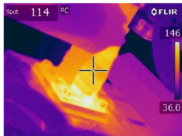
Figure 18: The temperature of the steam supply line to the heater
