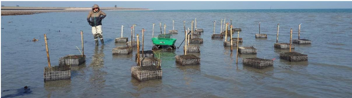
FIGURE 4, RANDOM PLACEMENT OF THE GABIONS WITH WOODEN POLES TO INDICATE THE LOCATION OF EACH GABION
