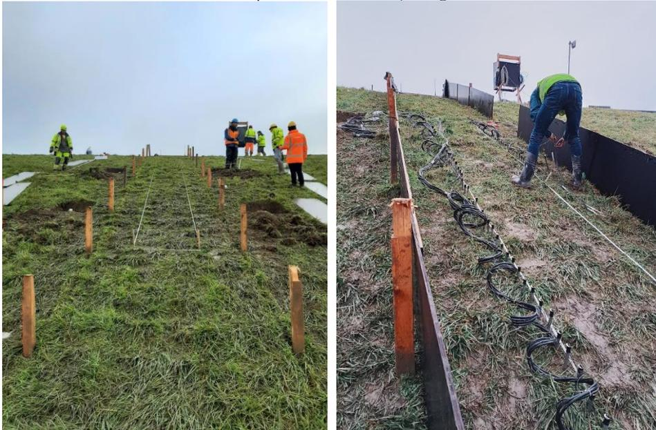
Figure 8.8. Left: Construction of the flume on section N-OF08 before installation of the ERT cables. Right: Installation of the ERT cables.
