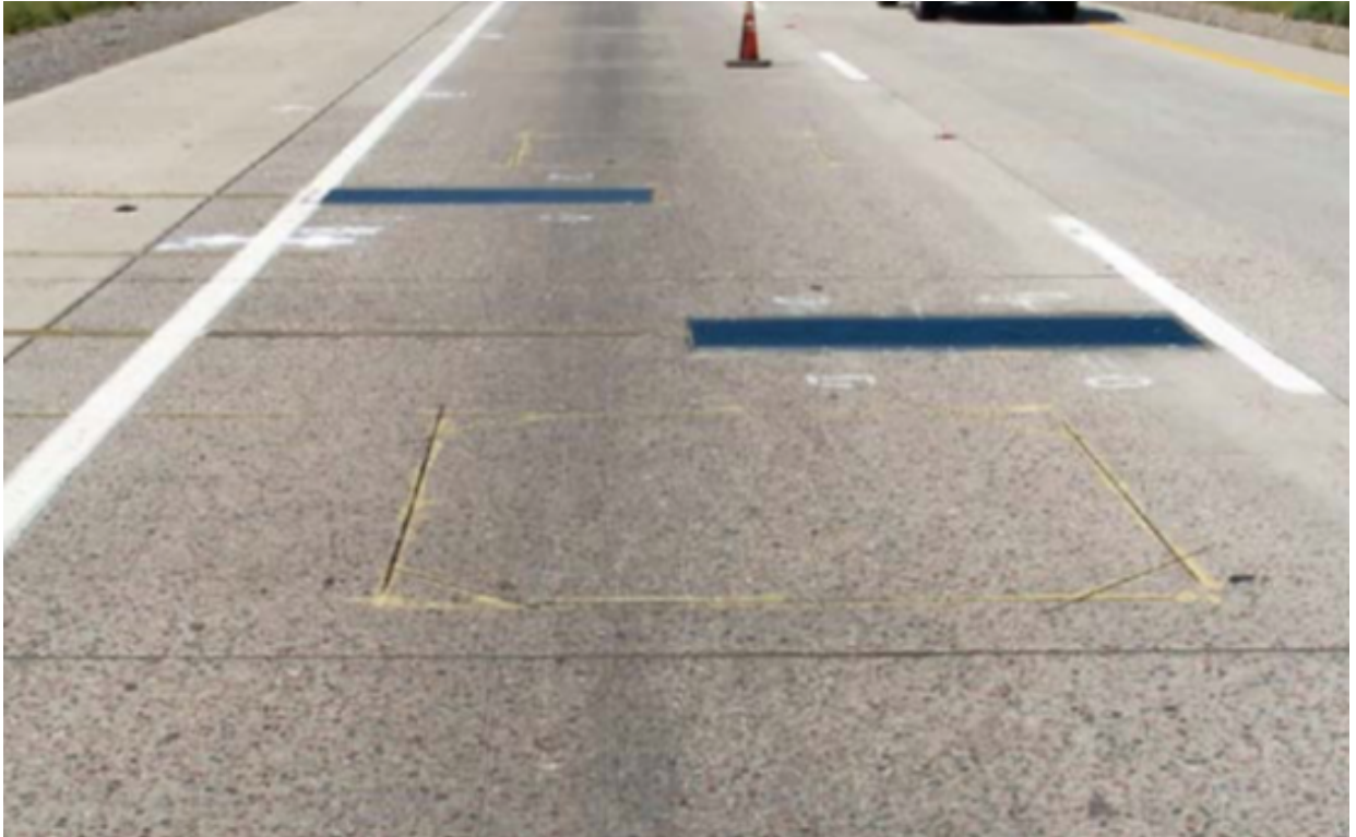
Figure 4. Plate sensor installation
