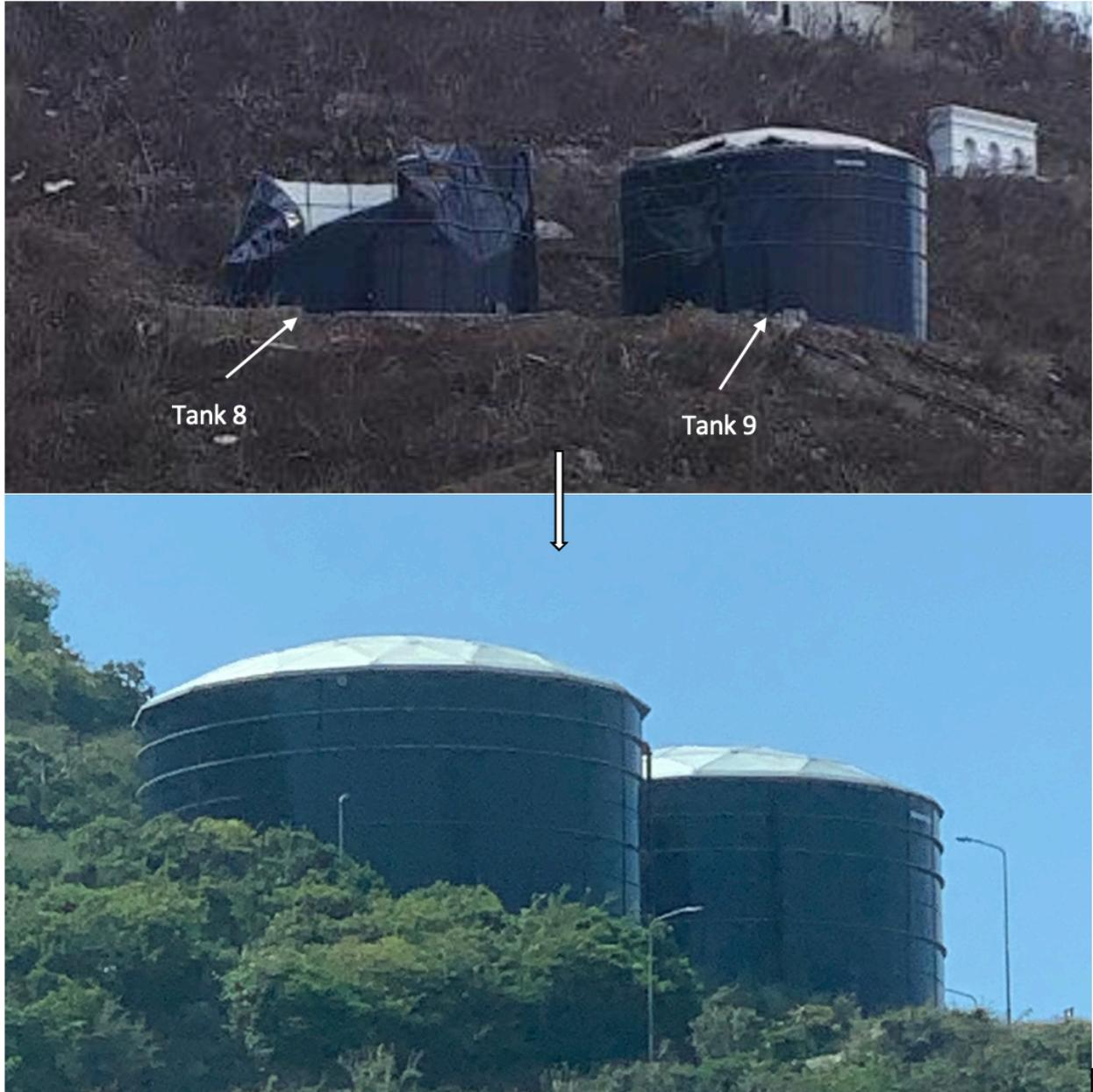
Figure 19: Point Blanche glass fused to steel water storage tanks after Hurricane Irma (top) and current picture(bottom). Made by Briana Halley using a picture from N.V. G.E.B.E staff and current picture taken by Briana Halley.
