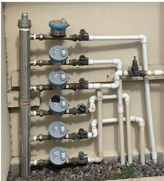
Figure 15: A Manifold with residential water meters. Taken by Briana Halley
