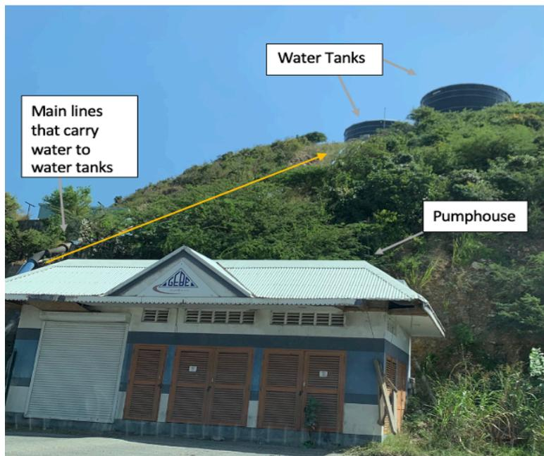
Figure 13: Point blanche location across Seven Seas water plant showing an example of the water distribution system of N.V. G.E.B.E. Taken by Briana Halley
