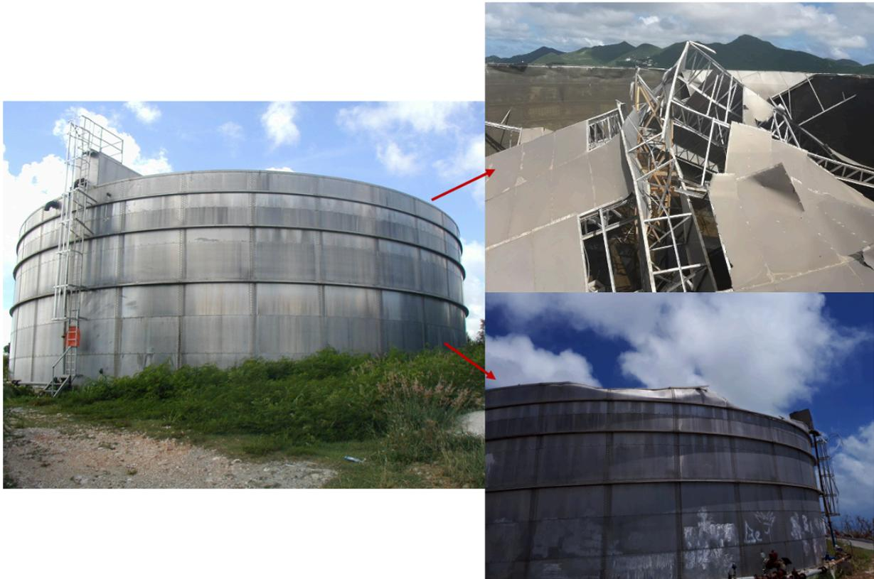
*Figure 20: Bolted aluminium sheet water storage tank in the district of Pelican Key before hurricane Irma (Left) and after the passing of the hurricane (Right). The dome of the tank as seen on the top right collapsed into the tank. Made by Briana Halley using photos provided by N.V. G.E.B.E. staff.*
