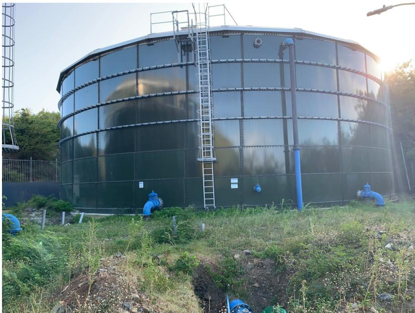
Figure 16: One of the glass fused to steel water storage tanks located in Cay Hill. Photo taken by Briana Halley, 2021
