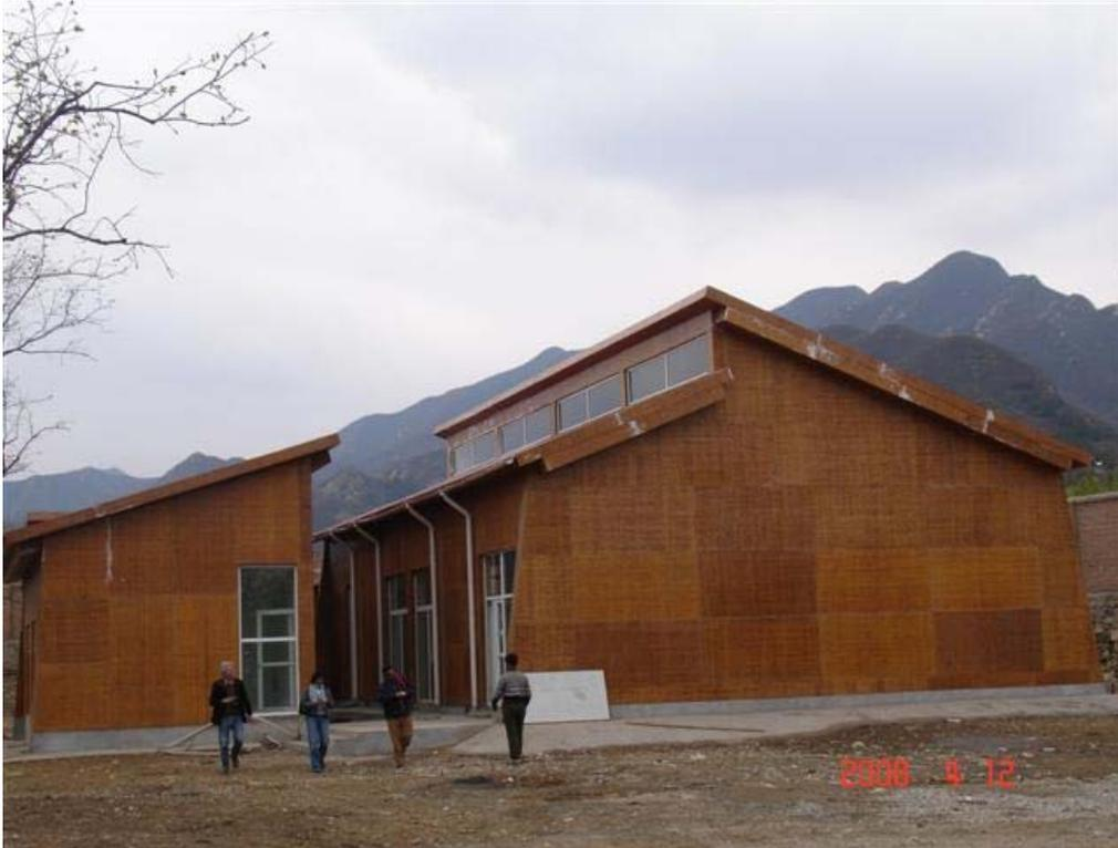
Modern bamboo housing in China. The cladding is made from woven bamboo mats, which are pressed into sheets. Source: Lou Yiping, INBAR (China)
