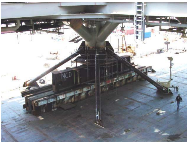
Figure 2.8 Photo of grillage and seafastening on a barge. The grillage beams will spread loads into the strong points of the barge.
