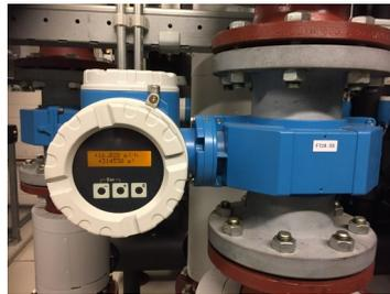
Figure 4.13 Flow sensor FT28-03
