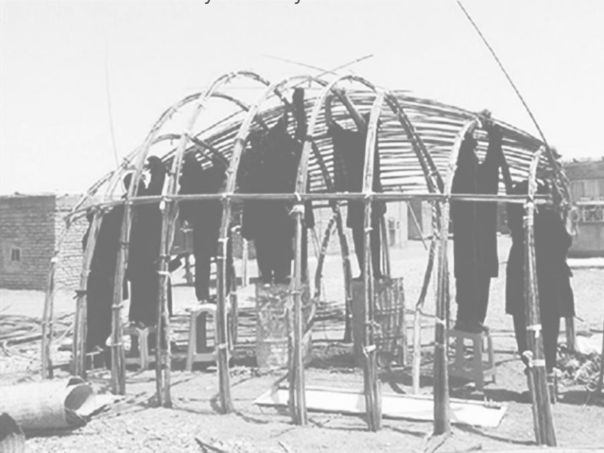
CAPAR is the traditional accommodation in Baluchistan fully made by Date timber
